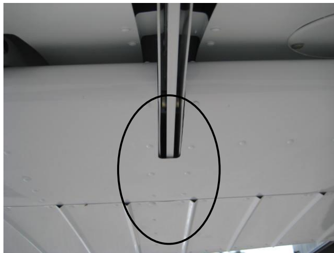
Figure 3: Outboard Flap Track Area of Particular Interest, Rib W.S. 118.0
